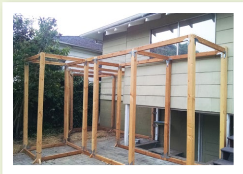
FRAMING IN PLACE
