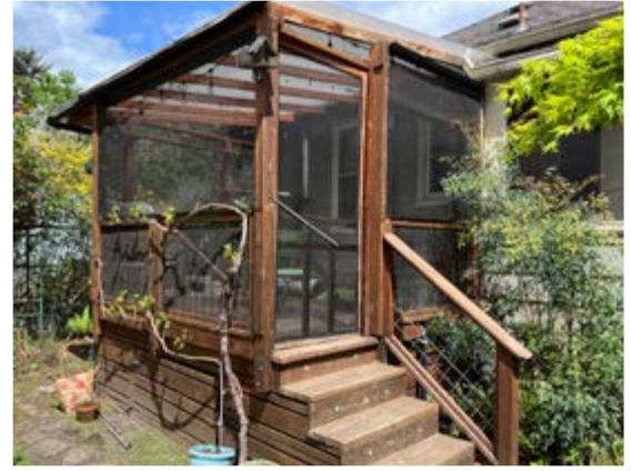
ACCESS FROM THE YARD
